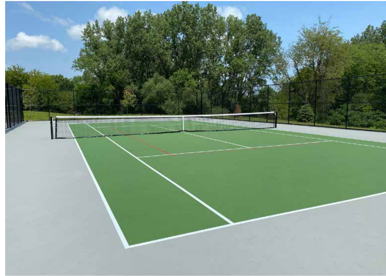
Combined tennis with pickleball court
